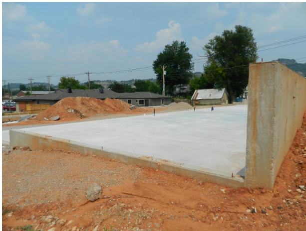
Construction continues on Carquest's new building on Main Street!
