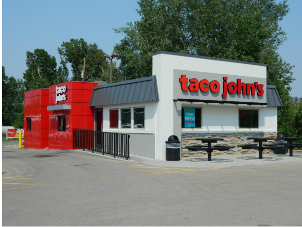
Taco John's has completed an exterior renovation and it looks great!
