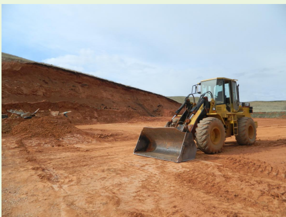
Continued Construction near Colorado Blvd.
